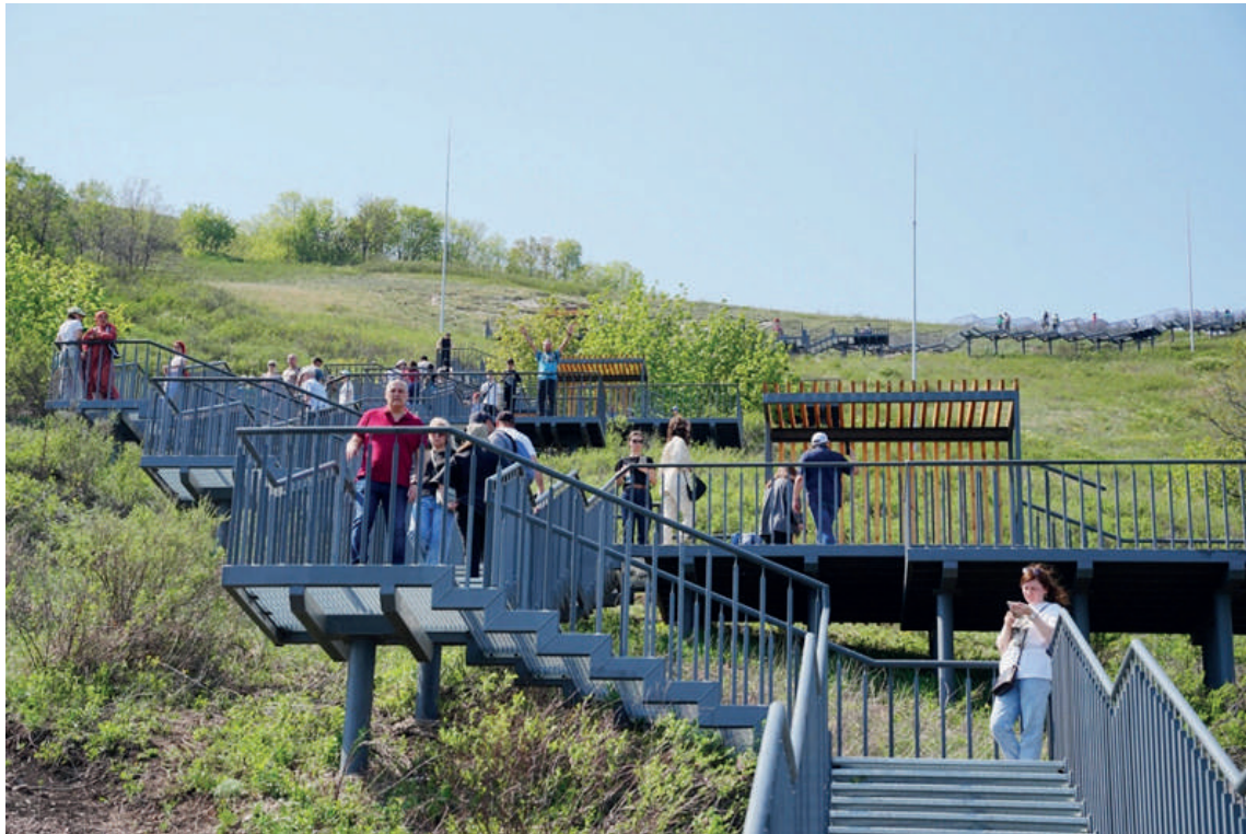
Fig. 63. Staircase on grief Toratau. Photo by A. Saitova.
